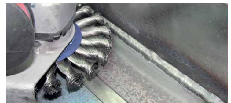
Cleaning of a welding seam using a knotted wire brush
