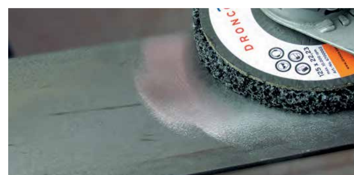
Cleaning and descaling of a steel surface using a coarse cleaning fleece
